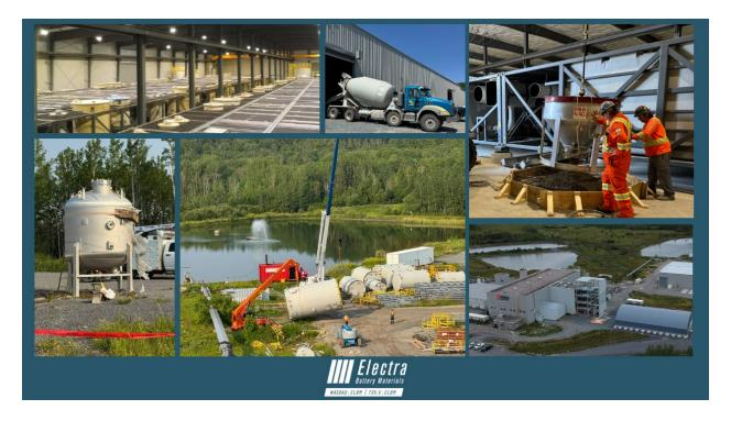
Key activities included concrete foundation work for SX tanks, installation of processing equipment, structural roofing, and upgrades to power, lighting, and septic systems. Engineering and procurement activities were also advanced to support readiness for full construction.
